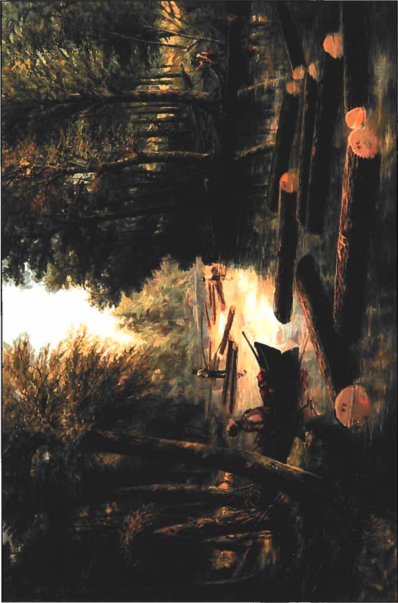
Clearing up the Deadheads. (1909) Many logs, usually referred to as "dead heads," went astray as they were being driven down the river to the mills on White Lake. They were forced ashore, stranded in shallow water, entangled in the roots of trees, and lost in the swamps. As shown here men are using their peaveys to drag deadheads back to the main stream. Notice that the logs have both end marks and side marks for identification. (James and Lois Rose, Montague)
