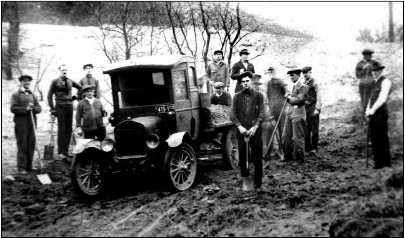
Road construction at Old Channel Trail
