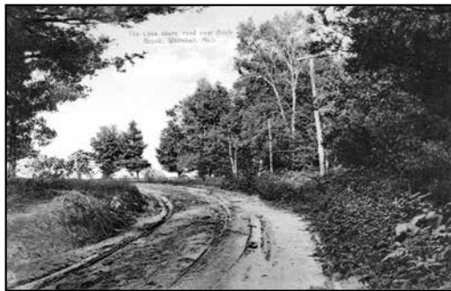
Another portion of the Lake Shore Road, near Birch Brook, shows how deeply rutted it was prior to paving. (Ogg Collection)
