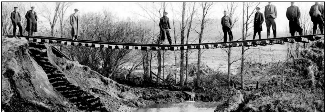
Another violent storm wiped out an earthen embankment over Happy Creek between New Era and Shelby that had once supported the Pere Marquette rail line. (Yakes Collection)
