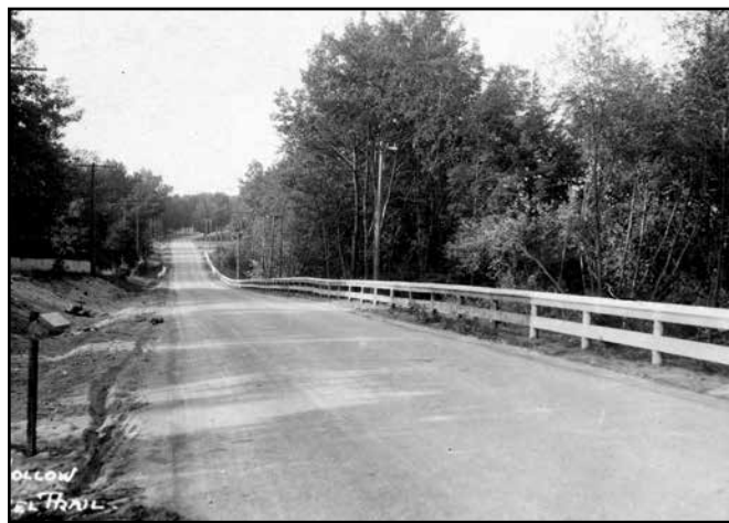
The road now known as Old Channel Trail, got its name when it was paved in 1923. The picture above is near Coon Creek. (Yakes Collection)
