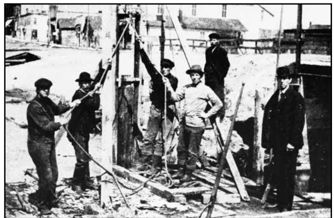
Work crews, such as this one, helped lay the drive the pilings that supported the causeway connecting Whitehall with Montague in the early twentieth century. (Montague Museum)
