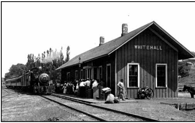
The Pere Marquette RR abandoned the Whitehall passenger depot, shown here, as well as the Montague depot, in 1926. (Yakes Collection)
