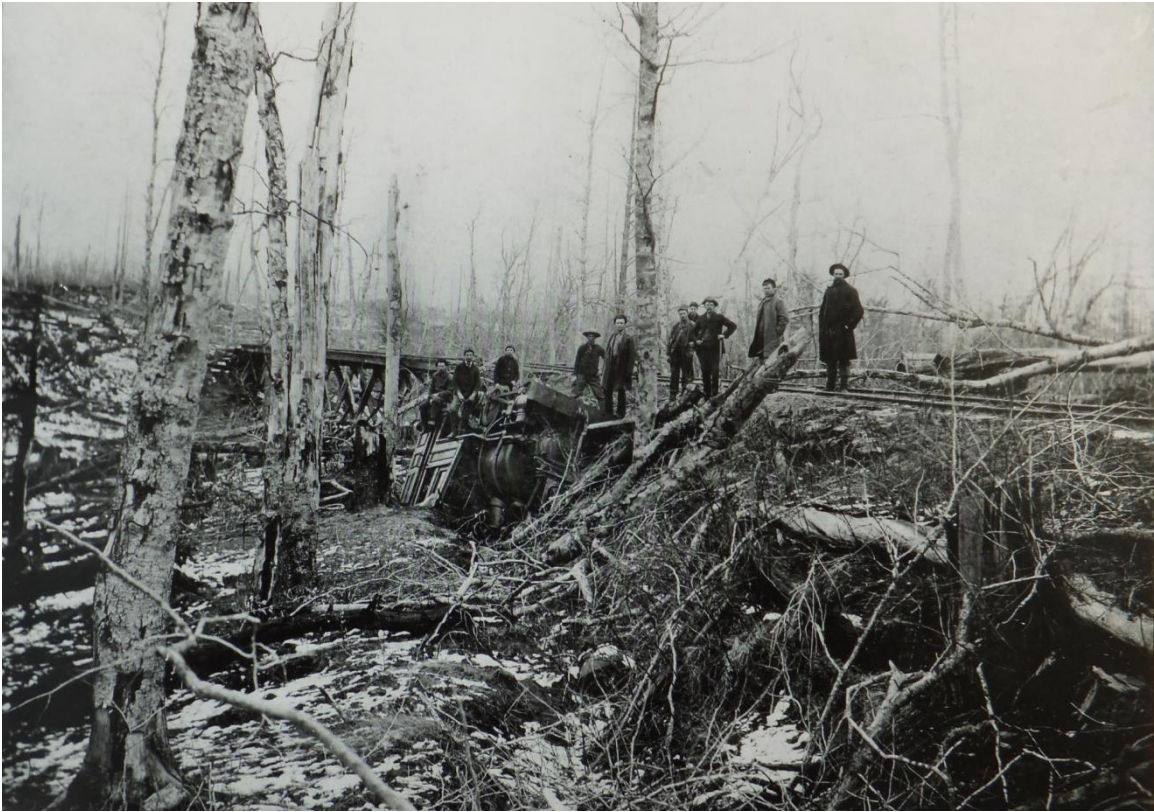
Figure 6. Train wreck photo showing the full trestle
