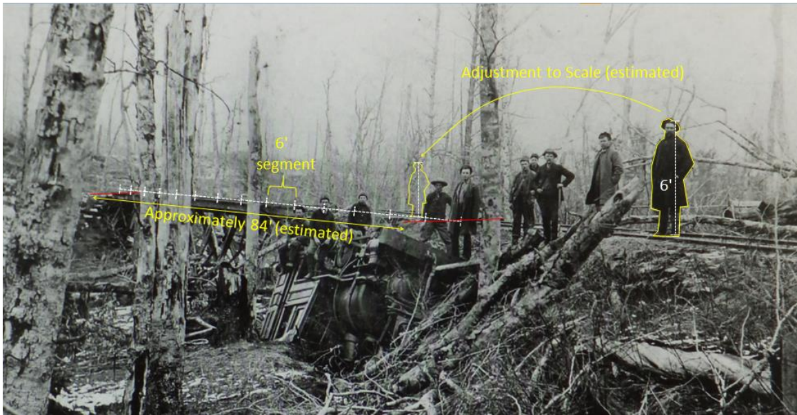
Figure 8. Scale estimation of the trestle length
