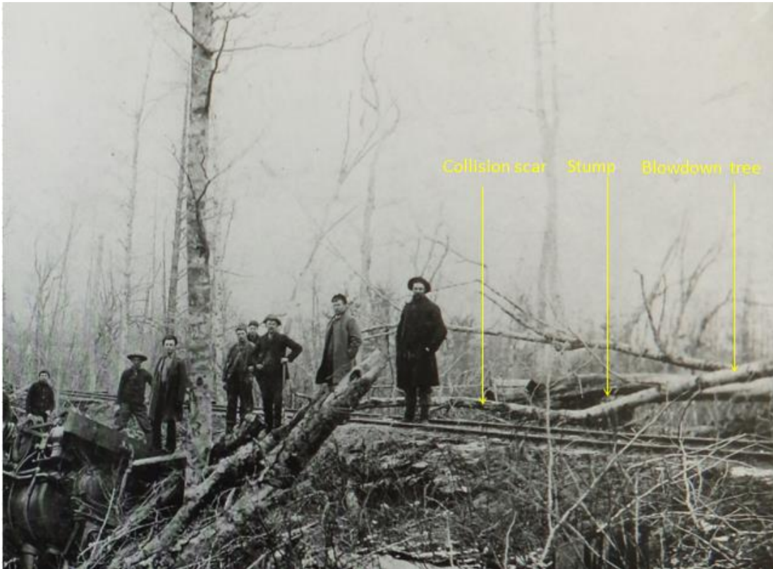
Figure 10. Train wreck photo with the stump and tree identified
