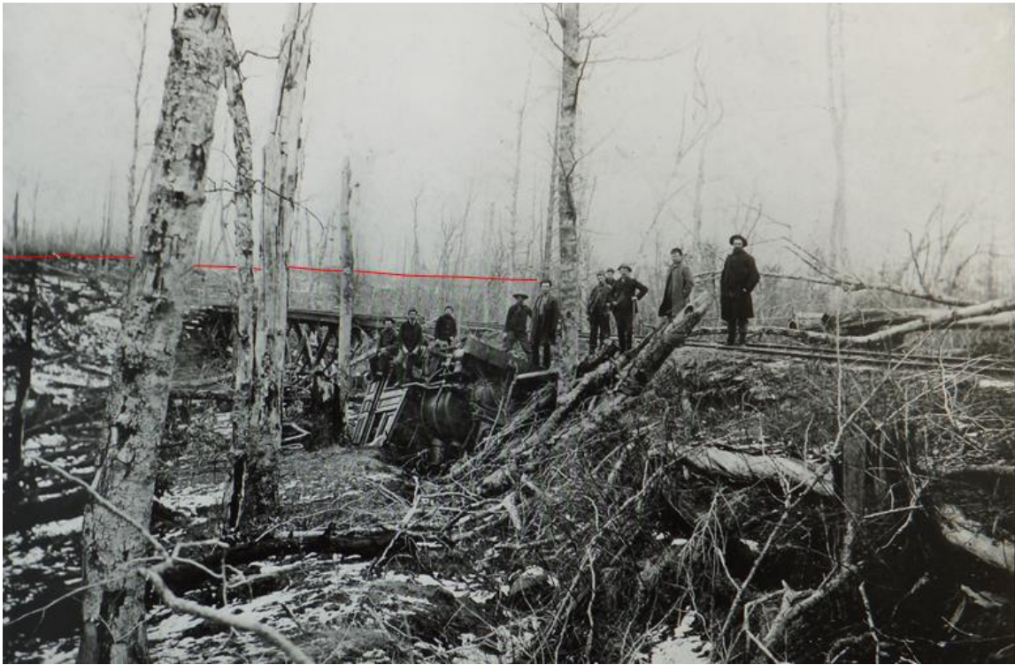
Figure 11. Train wreck photo with the background horizon identified
