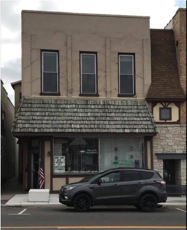
View of original bank building from a few years ago.
