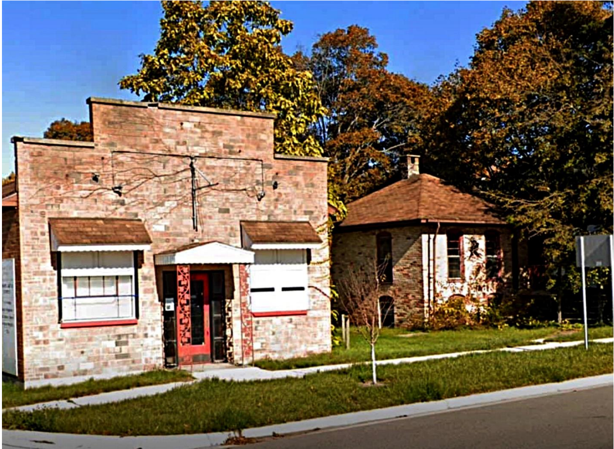
1938 Troy Laundry Building - located at 214 E. Colby
