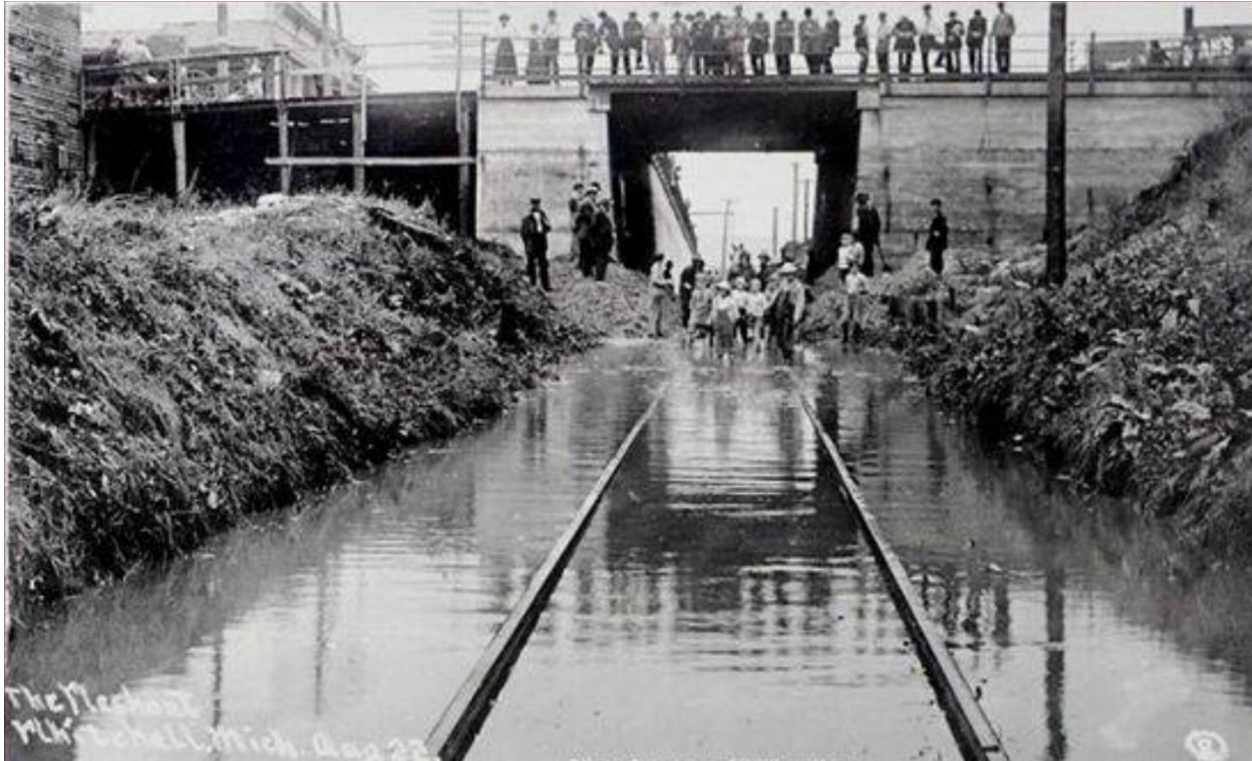
Railroad Tunnel Washout – August 22-23, 1910
