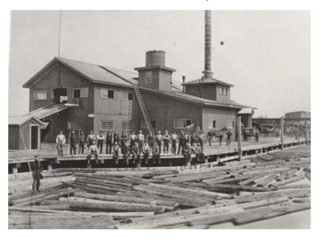
The Frank H. White & Co. steam mill as pictured was built around 1871-72 on wooden pilings on the Montague side of White Lake between Williams and Knudsen streets. It was a small mill with one circular upright saw and employed 40 men including C. Smith, engineer; John Ohrenberger, filer; J. Hulbert and G. Henderson, head sawyers. It was able to produce 70,000 feet of product in eleven hours. The mill operated until September 1888.
