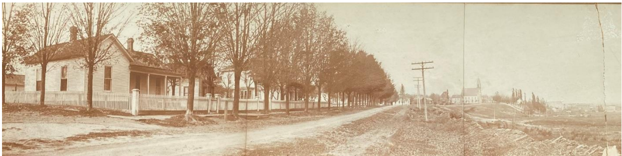
Figure 7. Old Channel Trail intersection with Richardson Street showing the compacted road bed awaiting the asphalt binder application
