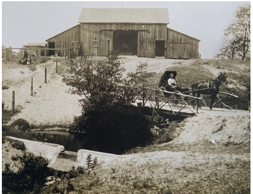
Figure 8. Bridge crossing and concrete dam on Buttermilk Creek circa 1915. Edmond Drumm property
