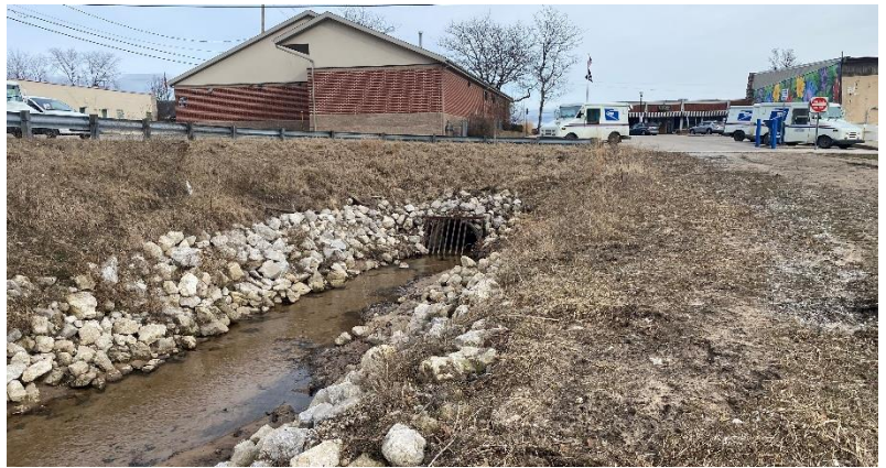
Figure 3. Buttermilk Creek entrance to underground passage beneath Montague
